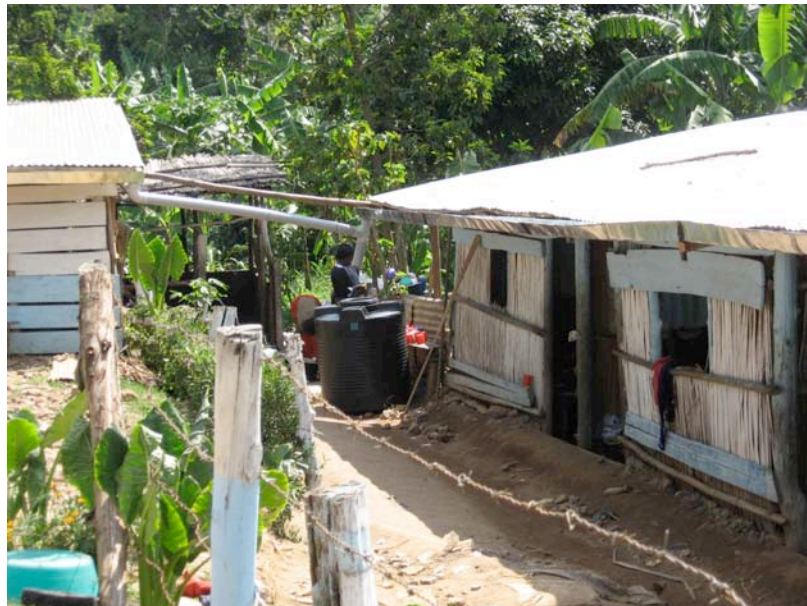
This shows some of the classrooms at Little Angels and the new rainwater catchment system.
