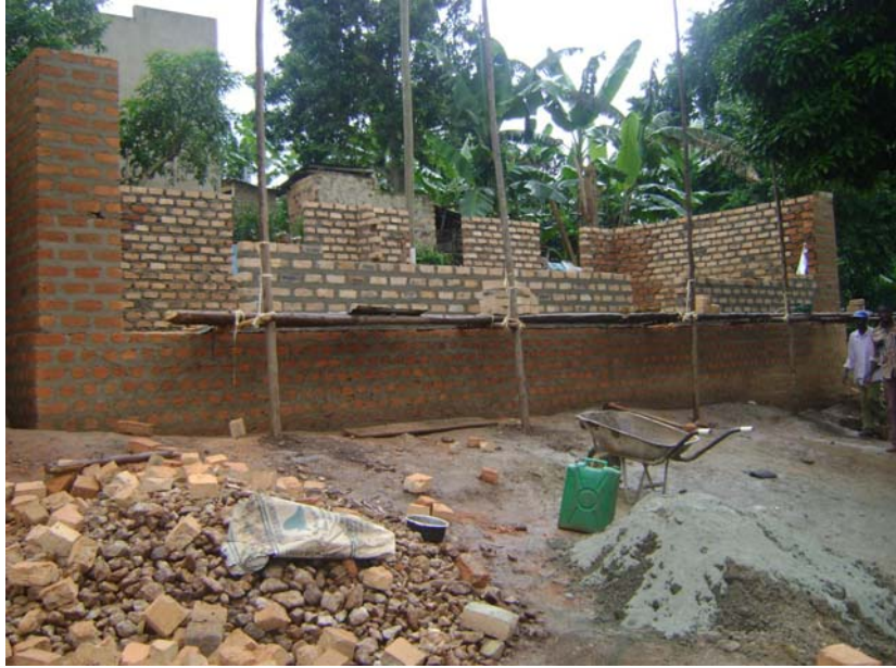
The foundation of the new classroom building at Little Angels
